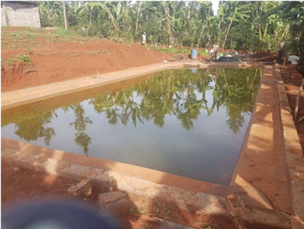
A water pond constructed in Kenya
