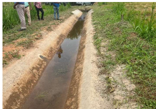
Water ways constructed in Sri Lanka
