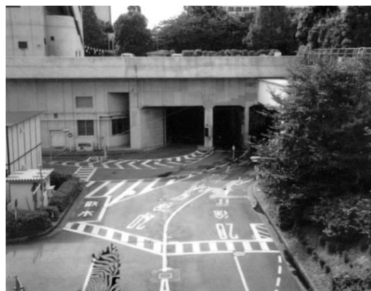
Photo 6-9 Underpass of Sugunami Incineration Plant (1982)
