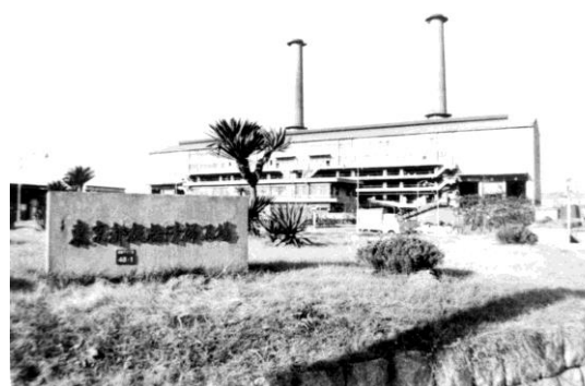
Photo 6-4 Itabashi Incineration Plant (Completed in 1961)
