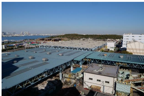
Photo 6-12 Overview of Incombustible Waste Treatment Facility and Bulky Waste Treatment Facility
