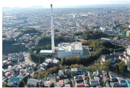
Photo 6-18 Ishinazaka Incineration Plant (130t/24h×3 unit)
