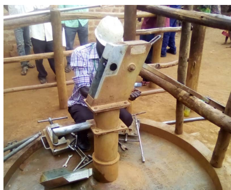
Photo 1 Repairing a Hand Pump
