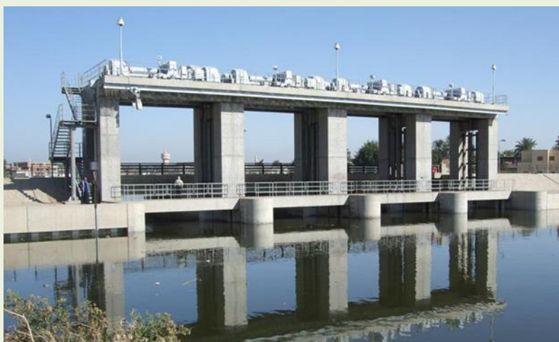
Monshat El Dahab Regulator on Bahr Yusef Canal (grant aid project for repair of the regulator completed in 2010)
