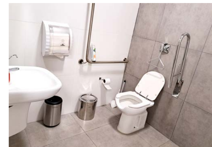
Barrier-free toilet at JICA Paraguay Office
