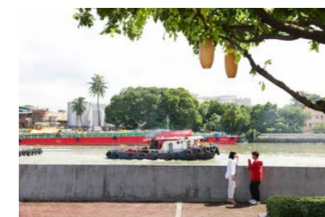
River embankment constructed under the Pasig-Marikina River Channel Improvement Project (Phase 2)
