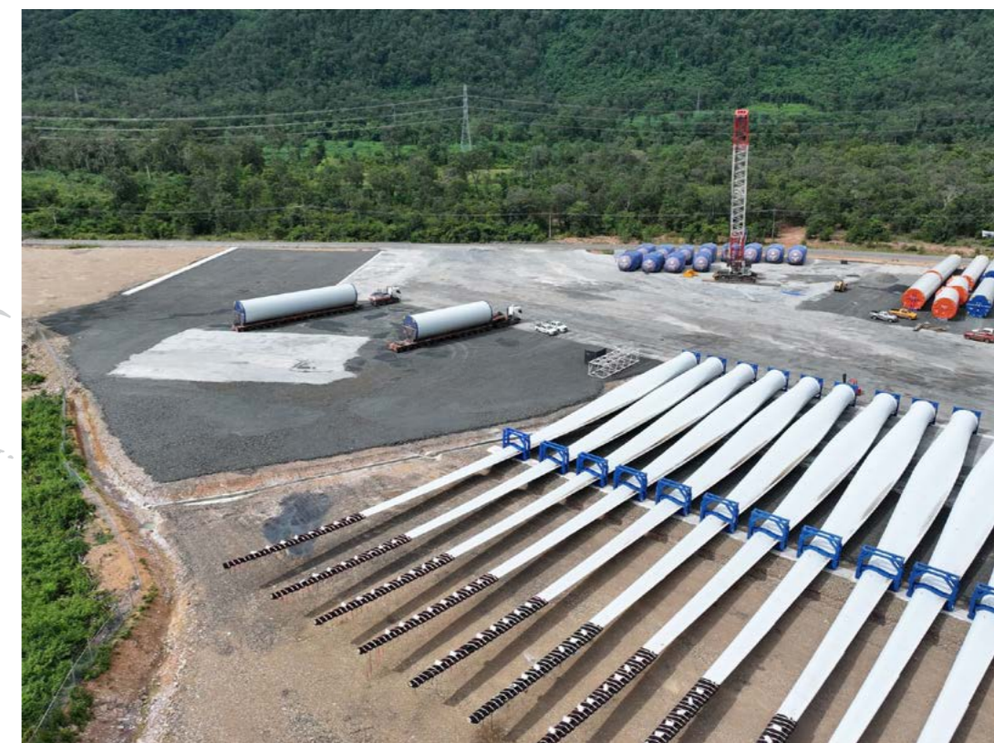
Wind power plant under construction
