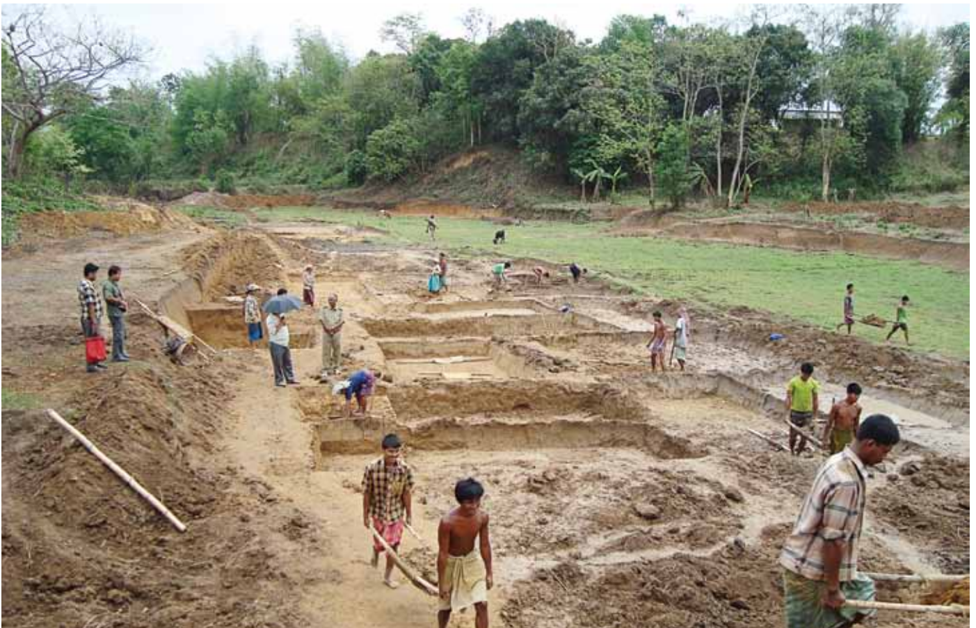
Soil & Water Conservation (SWC) Works by Jalema JFMC, Udaipur division
