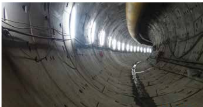
Completed Tunnel in Phase-II
