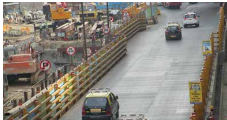
Construction work underway at the Mumbai Metro's Hutatma Chowk Station
