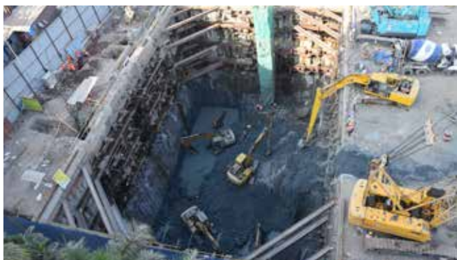
Aerial view of North shaft at Bandra Kurla Complex
