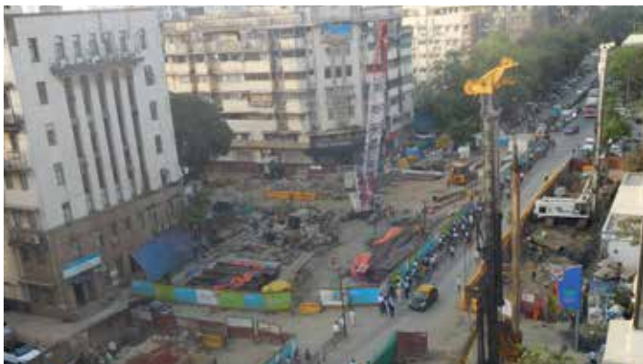
Bird-eye view of the Mumbai Metro's Churchgate Station
