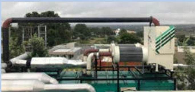
Investee Company of Neev Fund (II) : Pollution control devices on diesel gensets
