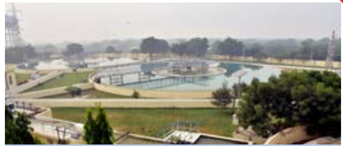
Water Treatment Plant under the Agra Water Supply Project
