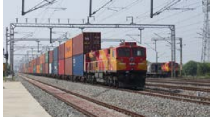
Western Dedicated Freight Corridor (DFC) Project links industrial, commercial areas and harbours between Delhi and Mumbai.
