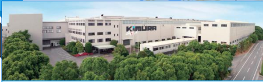
Omaezaki Foundry/Pattern Shop/ Machine Shop
