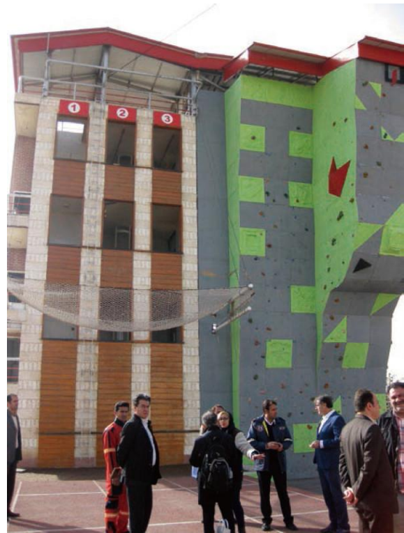
Firefighting training facilities constructed by former training participants
