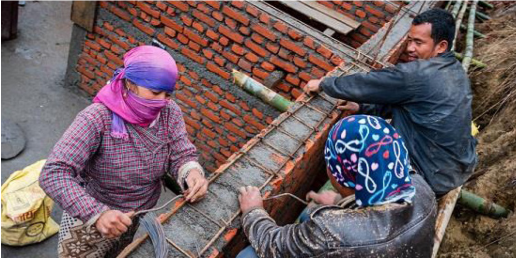
House owners constructing EQ resilient house .
