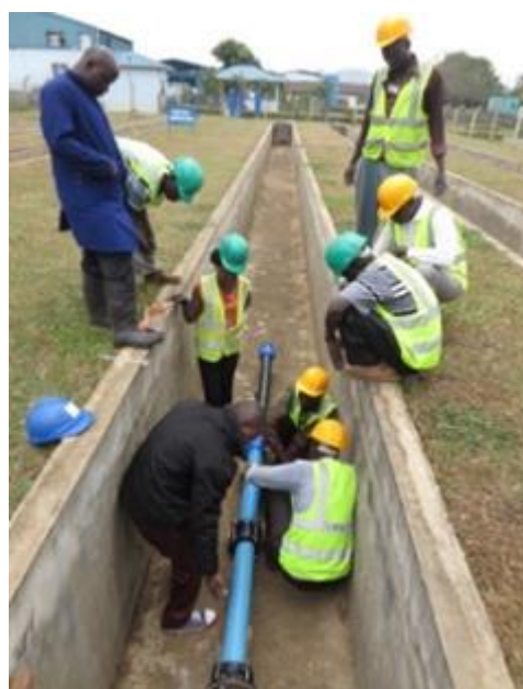
Photo 4 Pipe connection on demonstration site (Uganda)
