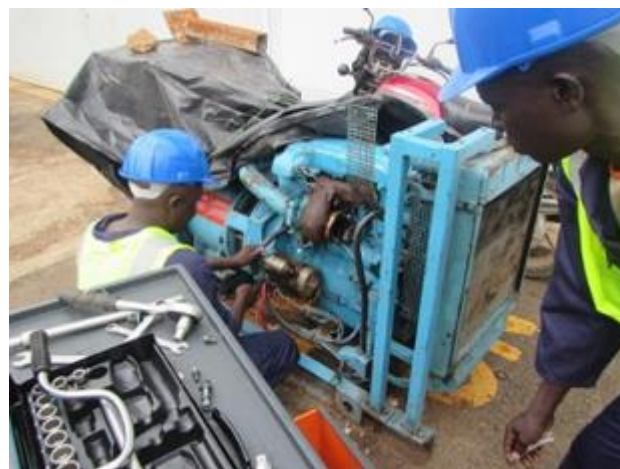
Photo 3 Electro-mechanical equipment maintenance (Uganda)
