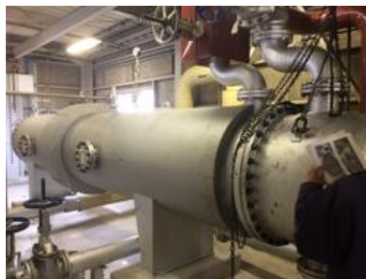
Figure 39 Heat Exchanger
