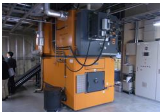
Figure 26 Boiler Used in the Biomass Village (made by Schmid, a Swiss company)
