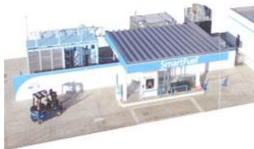
Figure 42 Hydrogen Station of the Shikaoi Hydrogen Farm
