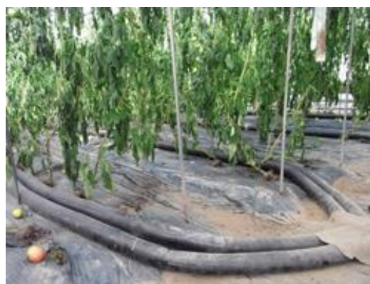
Figure 40 Pipes for Heated Water in a Greenhouse
