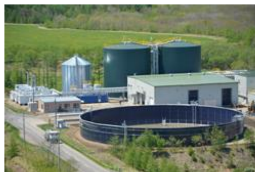
Figure 47 Betsukai Biogas Power Generation Facility
