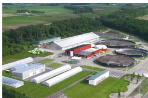
Figure 43 Shikaoi Town Environmental Preservation Center (Naka-Shikaoi)
