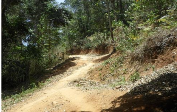
Newly opened feeder road
