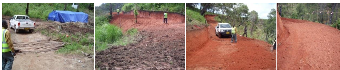
Well paved Road on Mountainous Terrain
