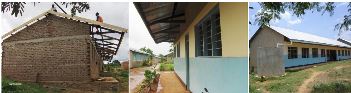
Classroom construction and rain water harvesting in Secondary schools
