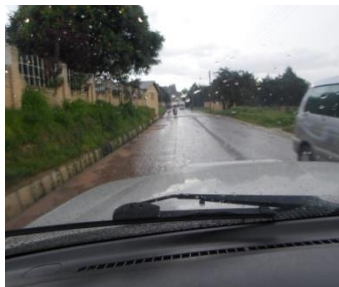
Tarmac road in Mafinga Town
