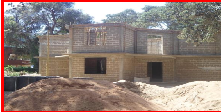
Tourist information center under construction through CLBT
