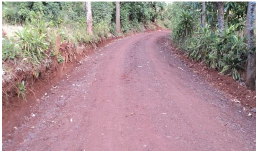
The road surface has been improved from slippery earth to gravel
