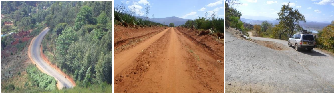
CLBT constructed double surface dressing, Earth and concrete roads
