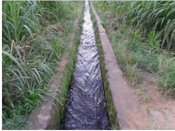
Irrigation canal at Siginali
