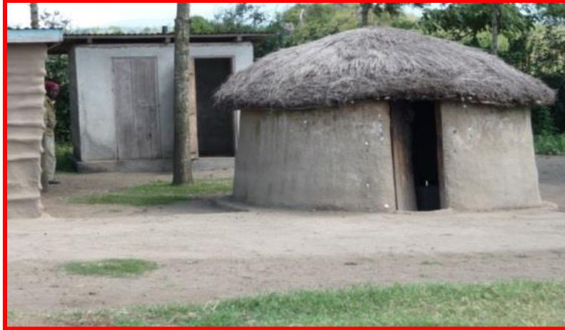
VIP toilet as seen from backyard
