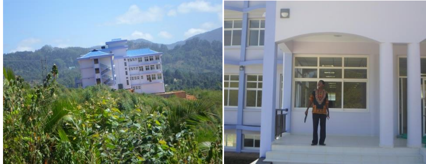
Newly constructed District Council office under close supervision of the Council engineer
