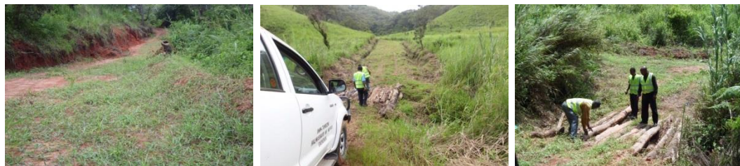
Construction activities in progress
