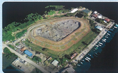
Palau M Dock Final Disposal Site (rendered with UAV imaging)
