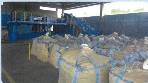
GUUN's Recycling Facility in Cebu
