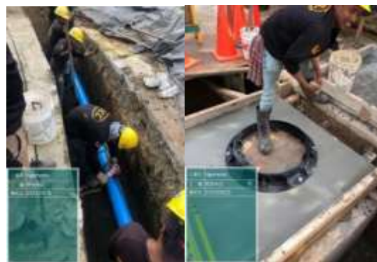
Figure 12 Pilot Construction (Pipe Renewal)
