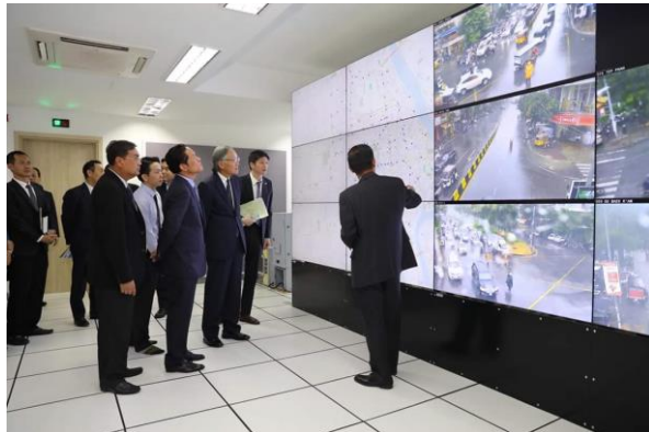
Traffic Control Center at PPCA
