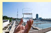
Water Supply Facilities of Phnom Penh Water Supply Authority
