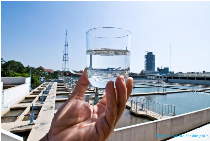
Water Supply Facilities of Phnom Penh Water Supply Authority
