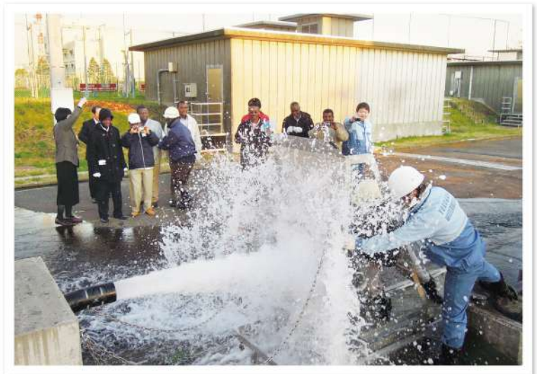
Participants from Africa observing water leakage repairs at a pipeline training facility
