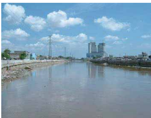
The improved western Jakarta flood-control canal
