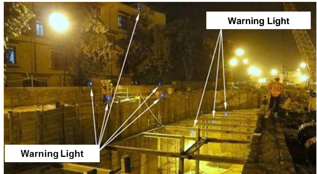
Construction site of AIIMS station of Delhi, where OSV was installed.
