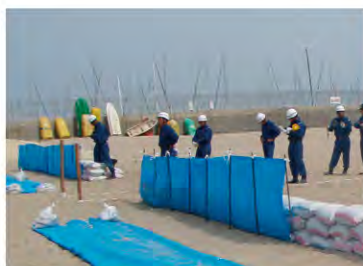
Sandbag Stacking with a Tarpaulin Wall
