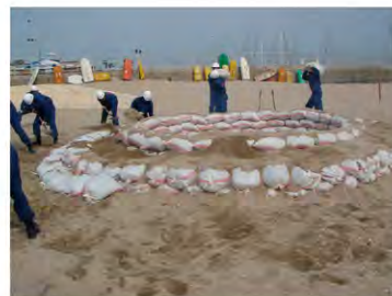
Sandbag Stacking in a “Stepped Pot” Shape
