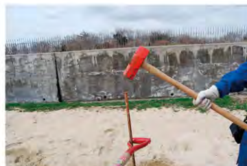
How to Drive in a Stake
