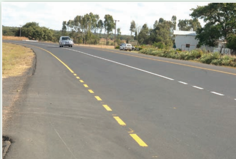
Building of new infrastructure
