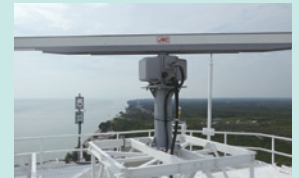
Sistem Radar (Foto: Japan Radio Company)
