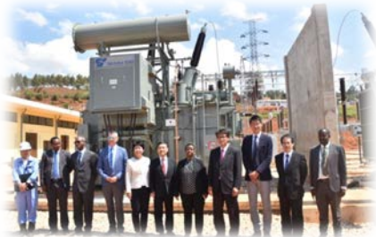
MININFRA and Japanese High officials at the Inauguration of Ndera Substation
