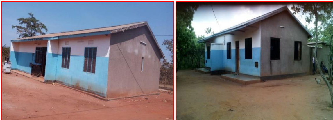
Nyakagwe Village Police Post and Staff House
