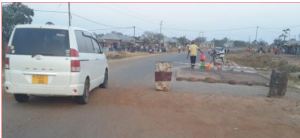
Construction of road humps to reduce accidents
