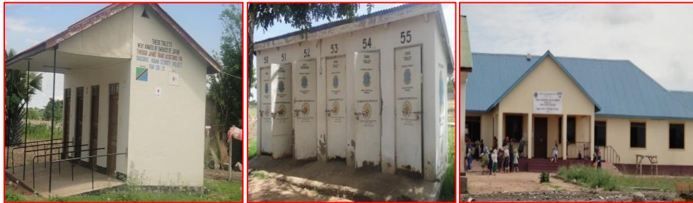
Toilets and Dormitories
