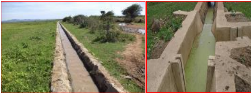
A lined trapezoidal canal and distribution points
