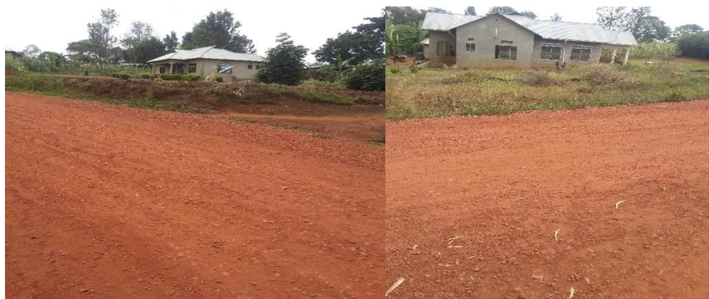
Improved residential buildings along the roads
