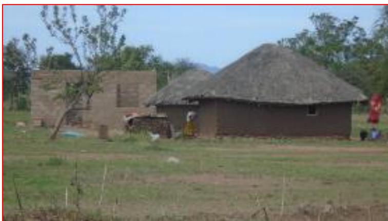
Ongoing construction of improved house and old house
