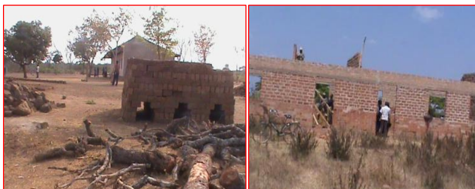
Bricks preparation and construction of satellite schools at Imalamawazo Butobela
