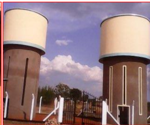
New Tank with 45,000lts and 90,000lts
