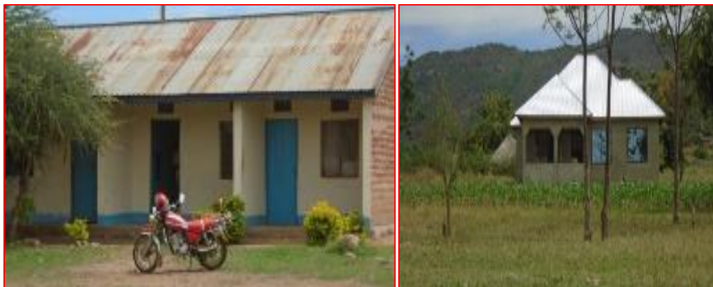
Improved houses, transport facility
