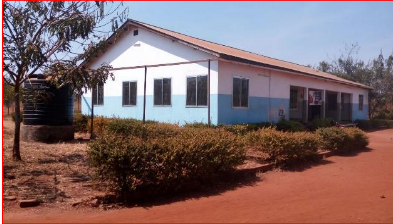
Nyakagwe Village Dispensary
