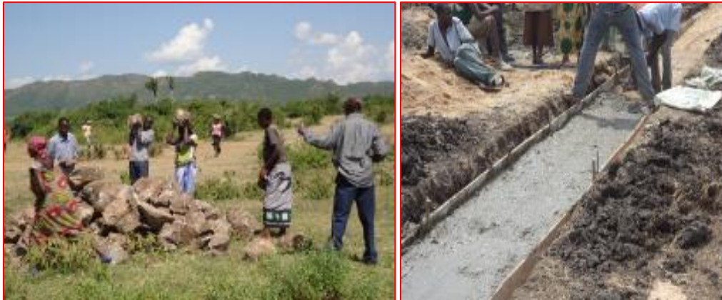
Farmers participating in construction of Canals
