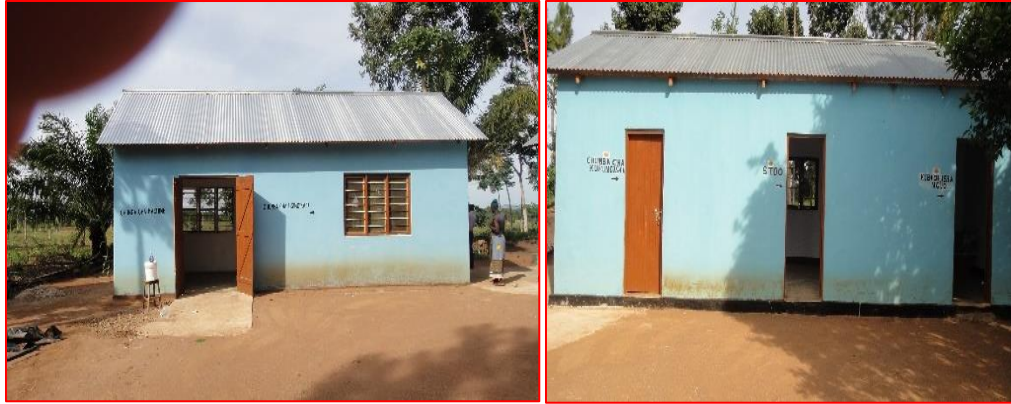
Cassava processing facility (machine house, store and change room)
