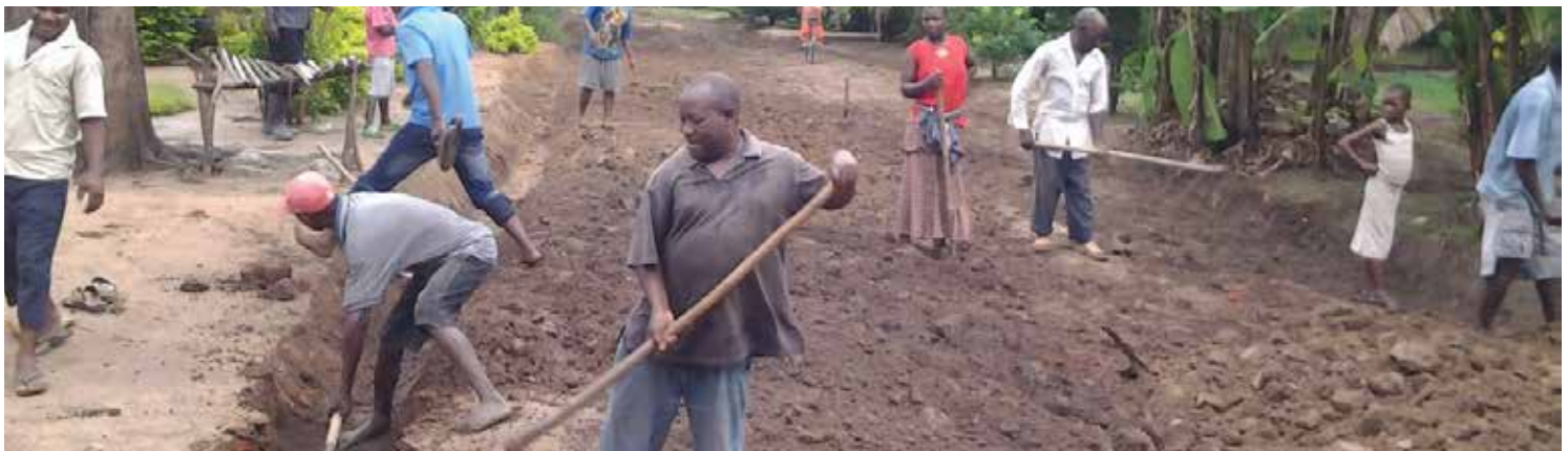
Villagers in Mang'ula B constructing Community Road by using O&OD methodology, which is “Self-Help Efforts” of the communities to deepen collaborative relationship between Local Government and Communities.
