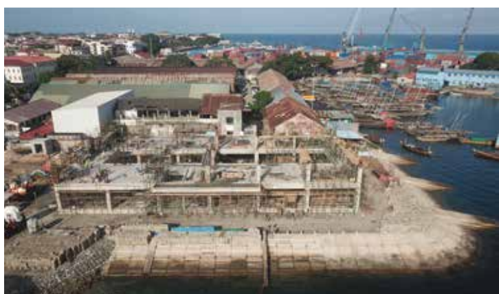
Construction of the Malindi Fish Market is in progress
