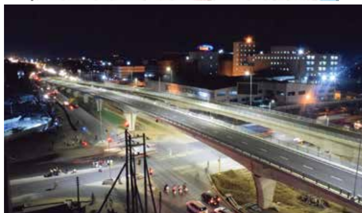
Improvement of Tazara Intersection
