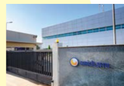
Unicharm Egypt Plant. Unicharm’s second plant in the Middle East after Saudi Arabia.
