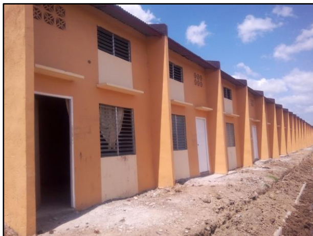
NHA relocation site in Pandi, Bulacan
