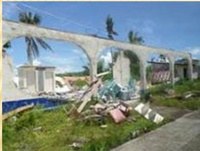
Damage after the Disaster
