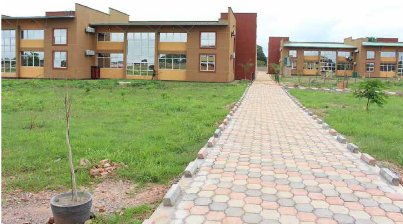
New facilities of National Science centre constructed with support from JICA. The centre has 16 labs. National Science Centre is a hub of national activities for science, mathematics and technology
