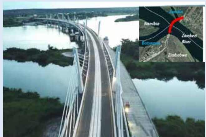
Kazungula Bridge and its Location
