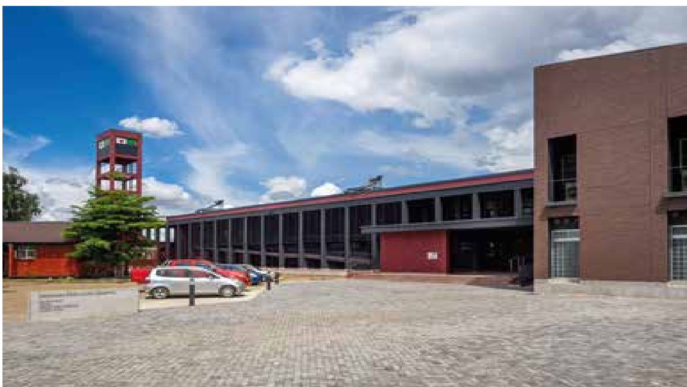
The three completed Hospitals in Lusaka (Kanyama, Chawama and Chipata 1st Level Hospitals)
