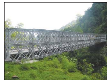
Current Loring Bridge
