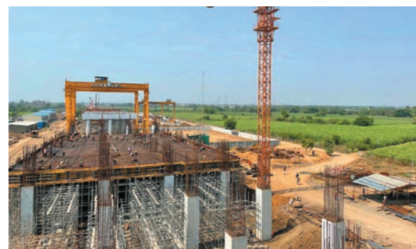
Construction is underway at Surat Station, one of the project sites.
