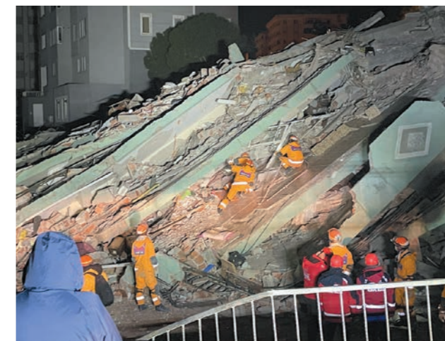
Turkey: The JDR Rescue Team conducted search and rescue operations while local residents looked on. The teams worked for seven days from the day after the quake hit.
