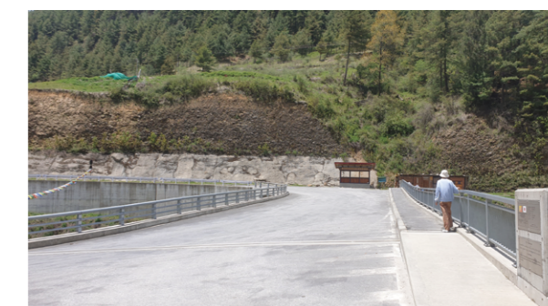
Nikachu Bridge with a sidewalk
