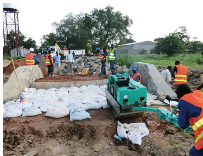
On-the-job training on repairs using sandbags for The Project for Capacity Development on Sustainable Road Maintenance and Management in Juba, South Sudan (September 2013)
