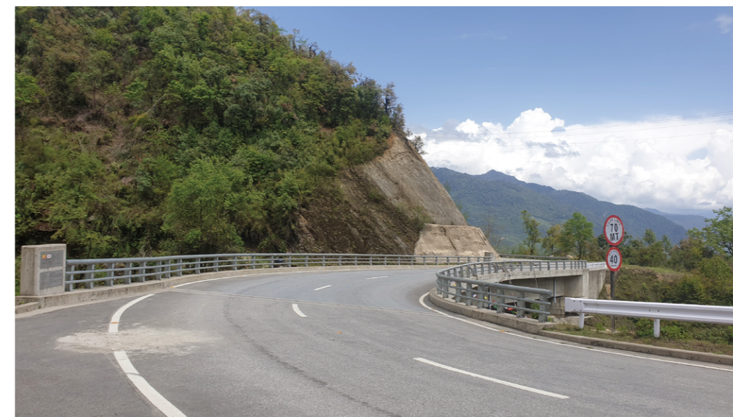
Curving Zalamchu Bridge
