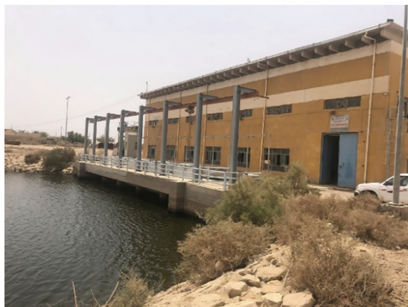
East Gharraf Drainage Pump Station
