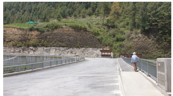
Nikachu Bridge with a sidewalk
