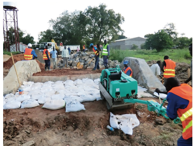
On-the-job training on repairs using sandbags for The Project for Capacity Development on Sustainable Road Maintenance and Management in Juba, South Sudan (September 2013)
