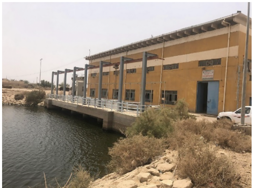
East Gharraf Drainage Pump Station
