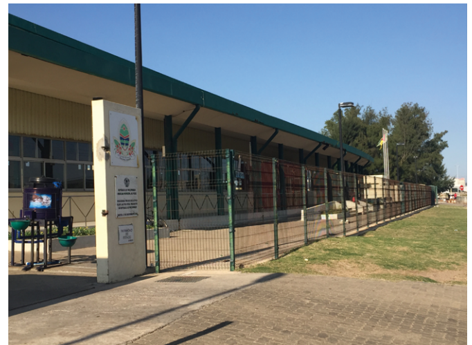
The exterior of Maputo Fish Market
