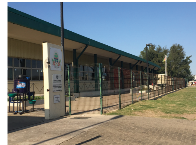
The exterior of Maputo Fish Market
