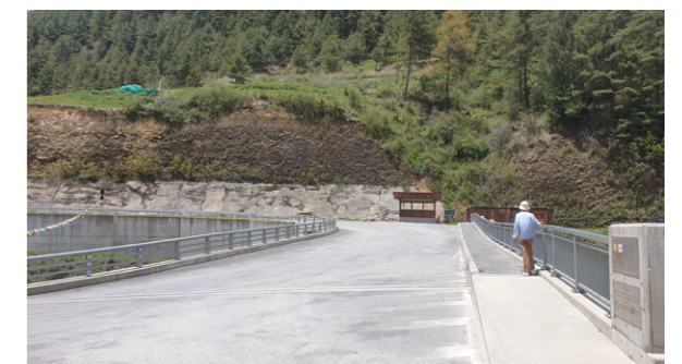
Nikachu Bridge with a sidewalk
