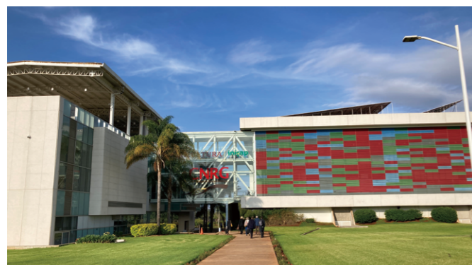
Exterior view of National Center for Genetic Resources (CNRG)
