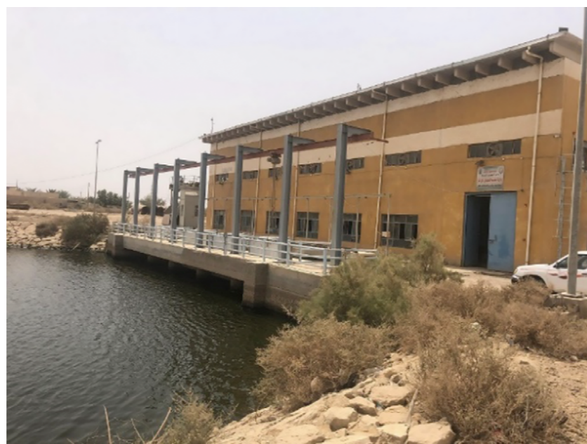
East Gharraf Drainage Pump Station
