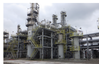
Natural gas production plant in Pertamina
