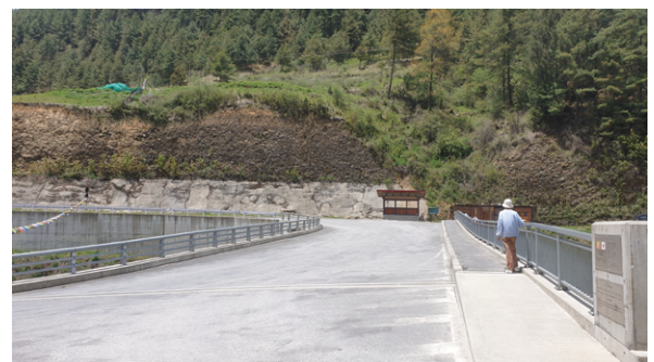
Nikachu Bridge with a sidewalk
