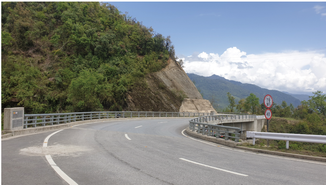
Curving Zalamchu Bridge
