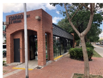
BRT Bus Station
