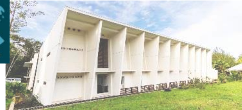
Pacific Climate Change Centre (PCCC) (Samoa) (Source : PCCC)
