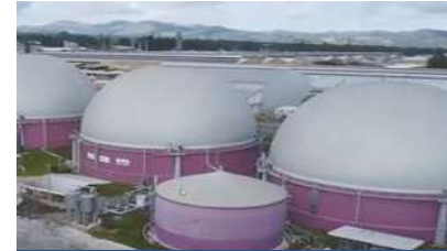
Biogas Power Generation, ITOCHU Corporation, Philippines
