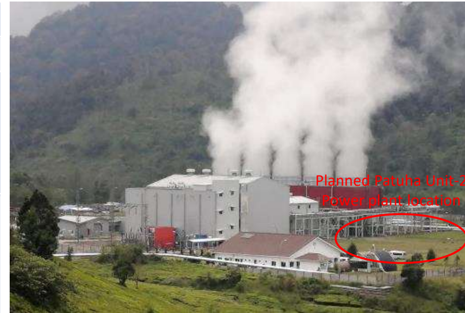
Patuha project site
