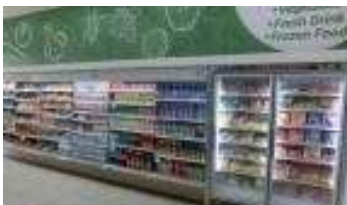
Energy saving at convenience stores, Panasonic, Indonesia
