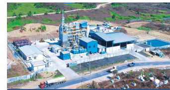
Waste to Energy Plant, JFE engineering, Myanmar
