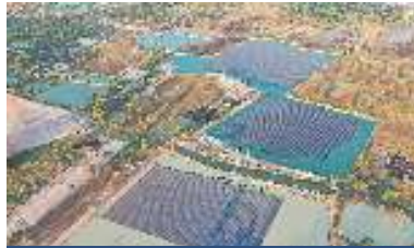
Floating Solar PV, TSB Co., Ltd., Thailand
