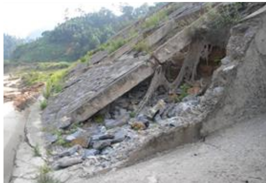
Situation of road slope collapse in Viet Nam and recurrence after countermeasures.
