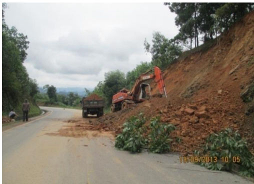
Situation of road slope collapse in Viet Nam and recurrence after countermeasures.
