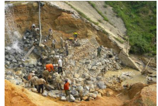
Situation of road slope collapse in Viet Nam and recurrence after countermeasures.
