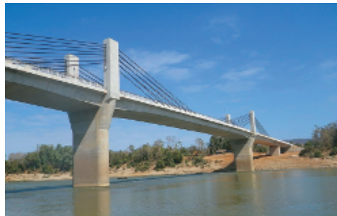
Laos: Sekong Bridge on NR16B completed in April 2018
