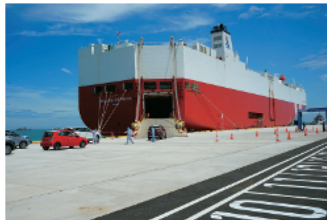
Indonesia: Some of the facilities at Patimban Port, where construction financed by ODA loans continues, were completed in December 2020
