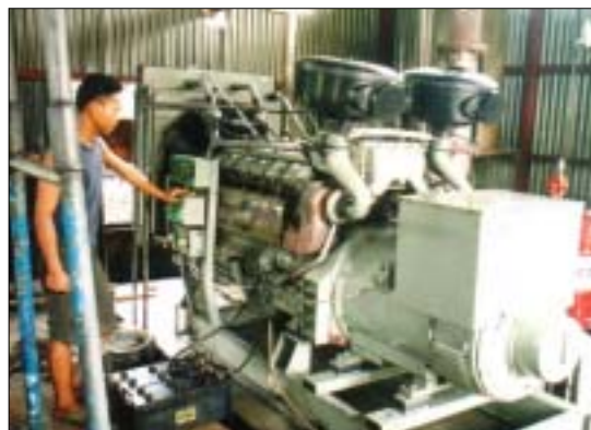
A Small Generator for Isolated Grid System
