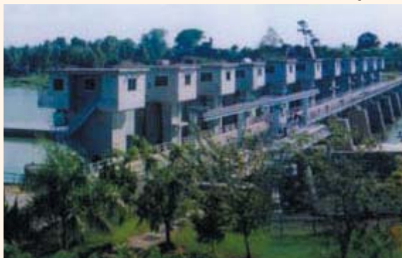
Komering-I irrigation facilities
