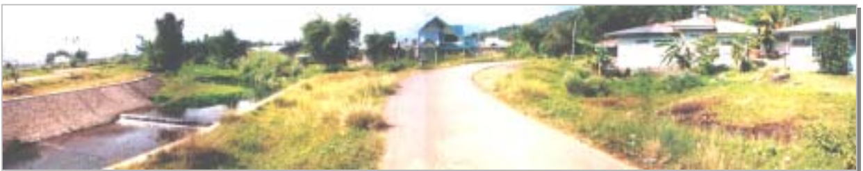
Figure 6 : Inspection road in Upper Jirak River
