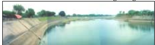
Upstream view at Lengkong Dam
