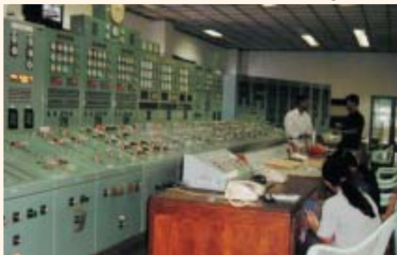
The control room
