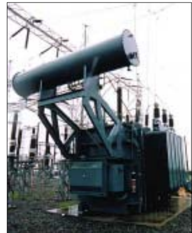
50 MVA Transformer
