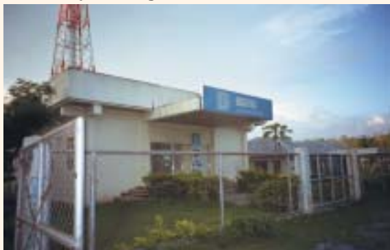
A telephone exchange
