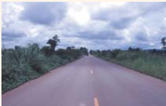
Improved roads under this project (near Udon Thani)
