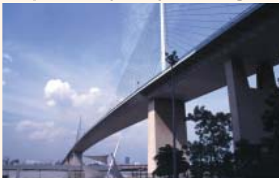
The cable stayed bridge crossing the Cha Phya River
